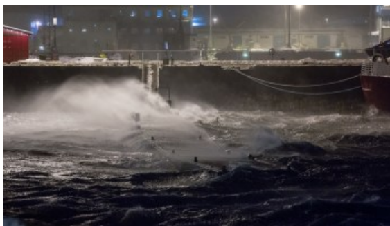
Iceland's Last "Oslo Tree" Badly Damaged By Storm
